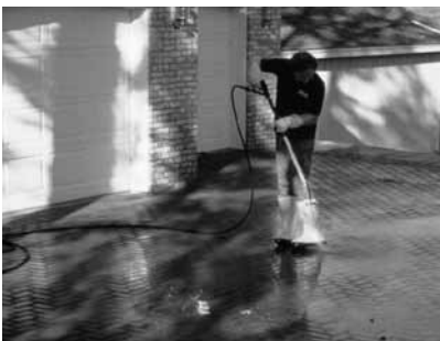
Figure 2. Pressurized cleaning equipment used by professional cleaning and sealing companies can bring out the best appearance from pavers.
